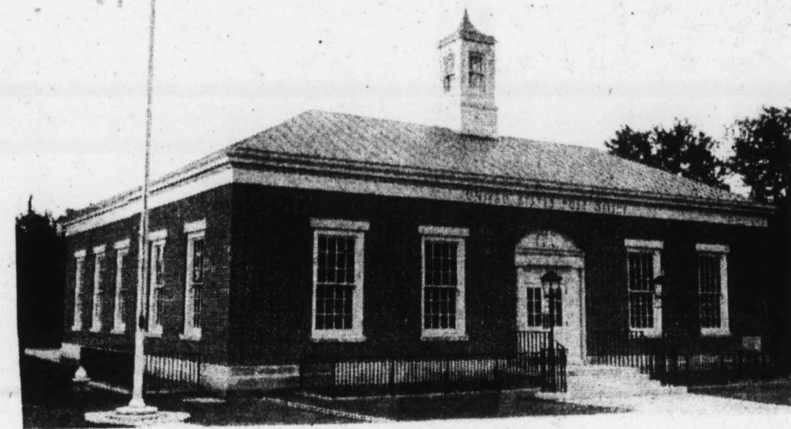
RIPLEY POST OFFICE built in 1937. Addition was added early 1960's.
